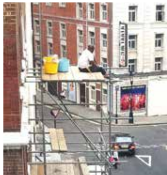
Sitting on a scaffold with no guard rails, harness or other measures in place.
