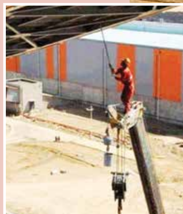
Sitting on a scaffold with no guard rails, harness or other measures in place.
