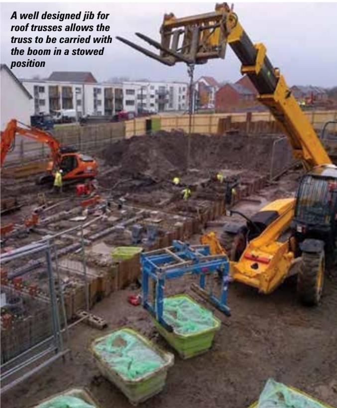
lifting and travelling with suspended loads is generally more hazardous than lifting unit loads on the telehandler's forks.
