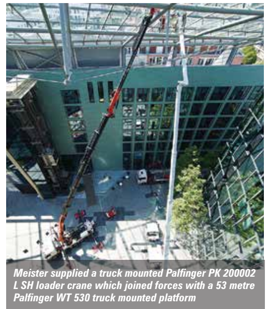
The PK 200002 was extended 38 metres and using the vacuum lifter, removed the defective pane
