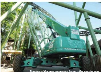
Erection of the new generation hyper roller coaster was helped by a 180ft Genie SX-180 and 85ft S-85 boom lift
