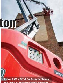
A new 63ft SJ63 AJ articulated boom was used to restore several sections of brickwork with traditional lime mortar at Laughton Place, a 16th century historic site.
