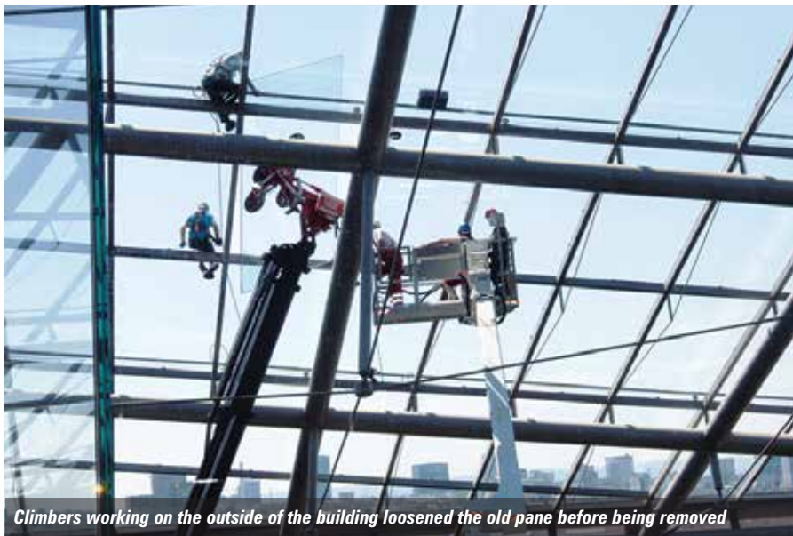
The PK 200002 was extended 38 metres and using the vacuum lifter, removed the defective pane
