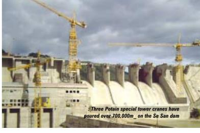
The MD 900B worked with a 60 metre jib, which provided 13.1 tonnes lift capacity at its tip. It was equipped with a six metre bucket allowing the crane to pour between of 80 and 100 cubic metres of concrete an hour.
