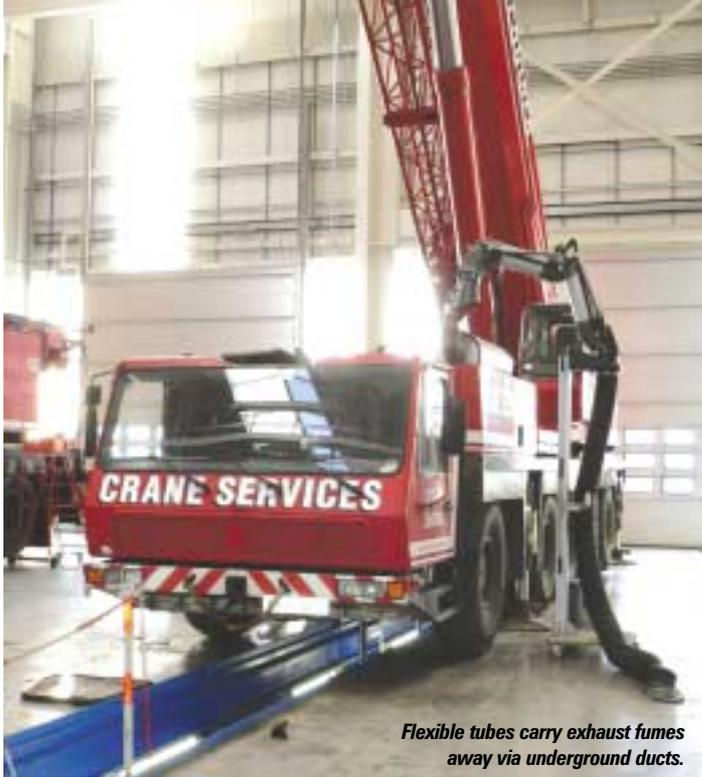
*Flexible tubes carry exhaust fumes away via underground ducts.*
