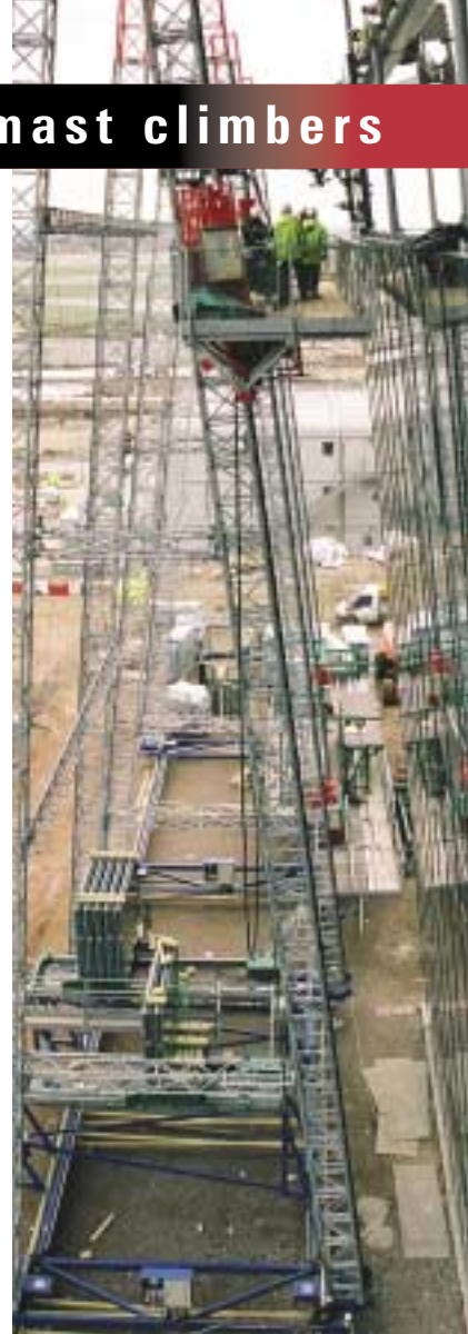
The solution to the access and lifting problem was solved with a twin mast A-Frame.
