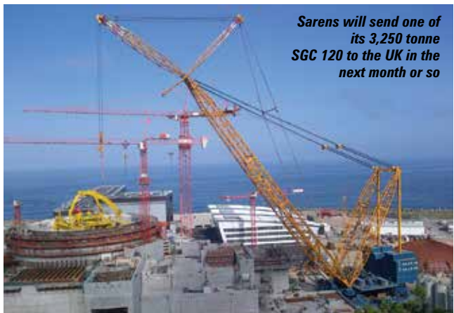
ALE's new modular design 3,400 tonne capacity heavy-duty jib has lengths of up to 100 metres
