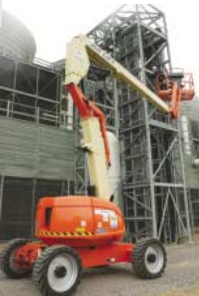
External maintenance of enclosed cooling tower pipe-work at Didcot Power Station.
