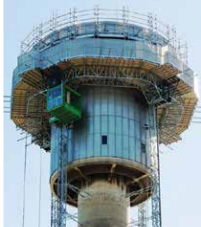
A circular demolition platform in Sydney
