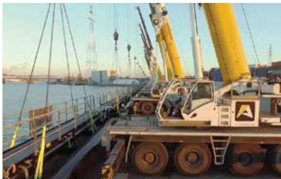
Each crane lifted a 6.1 tonne section of pipe.
