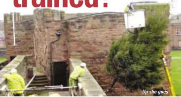
This is a very unusual incident, on the one hand one of the worst pieces of machine abuse is taking place, the operator is using the platform to lift a suspended load. As if that is not bad enough, it is a load of an unknown weight and is attached to the worst possible point, the thin finger guard rail which is not only the furthest distance from the centre of rotation, but also as it is attached to a plastic bucket, hardly likely to be strong enough!
