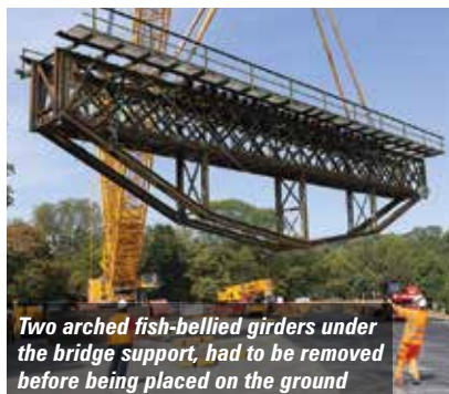
The LR 11000 with 96 metre main boom removing the 60 tonne bridge
