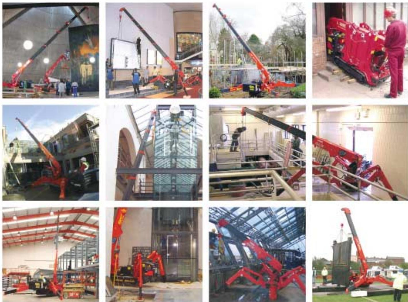
The new **UNIC** range of mini-crawler cranes. Discover incredible power and reach in the most confined of working environments. With an overall width from 600mm, **UNIC** mini cranes are small enough to get in there, and big enough to get the job done.
