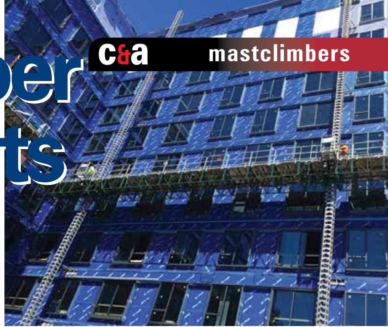
A twin masted, twin platform mastclimber
