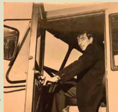
The early Days Meade at the controls of a crane.
