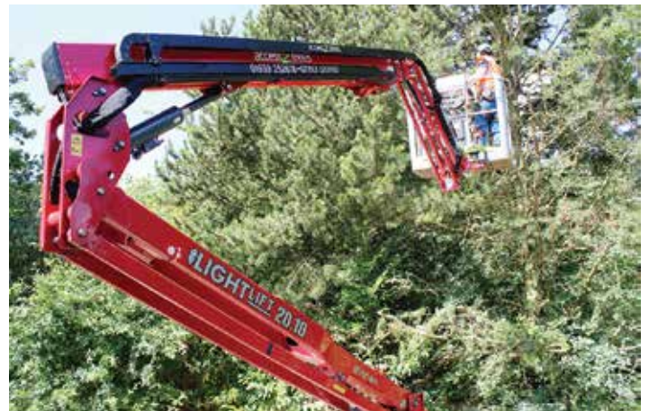
Dangerous as tree work is, it is far safer when carried out from an aerial work platform rather than actually climbing the tree
