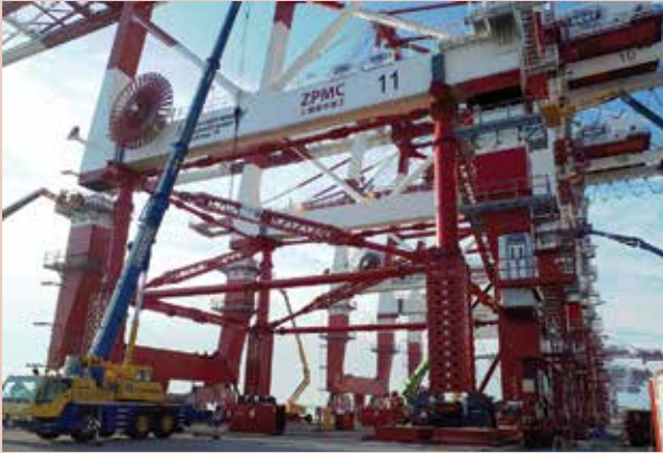
The Mega Jack 800 has 800 tonnes capacity in each of the four towers and performed the jacking in 12 stages.
