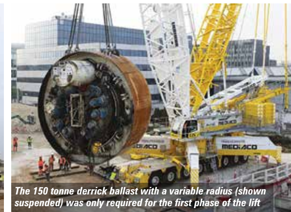
The disc cutter with hydraulic drive measures almost eight metres in diameter
