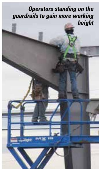
Operators standing on the guardrails to gain more working height
