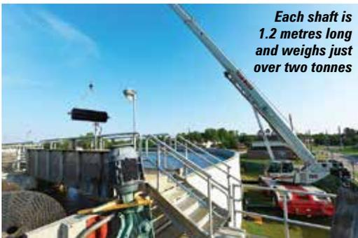
Each shaft is 1.2 metres long and weighs just over two tonnes
