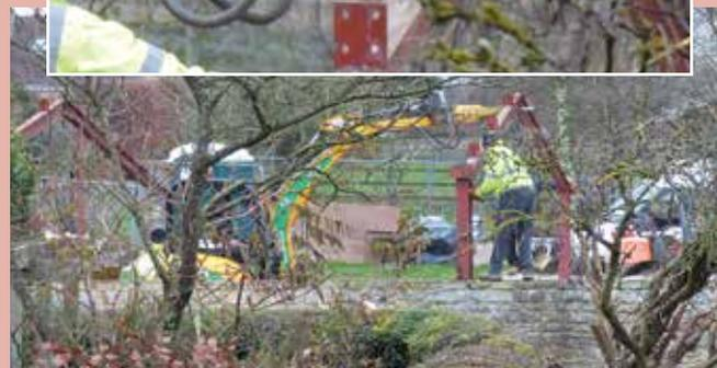
Spotted in the UK a demolition contractor dismantling a steel frame building using an excavator and breaker for all the lifting. As they removed the bolts from the joined roof truss, it rotated on the breaker tool wildly, almost knocking one of the men in the head and brushing the other off the wall he was standing on.
