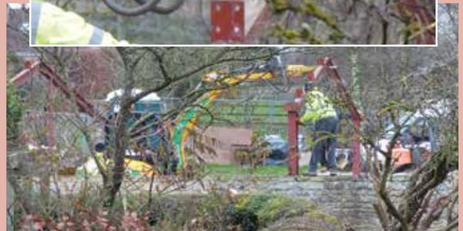
Spotted in the UK a demolition contractor dismantling a steel frame building using an excavator and breaker for all the lifting. As they removed the bolts from the joined roof truss, it rotated on the breaker tool wildly, almost knocking one of the men in the head and brushing the other off the wall he was standing on.
