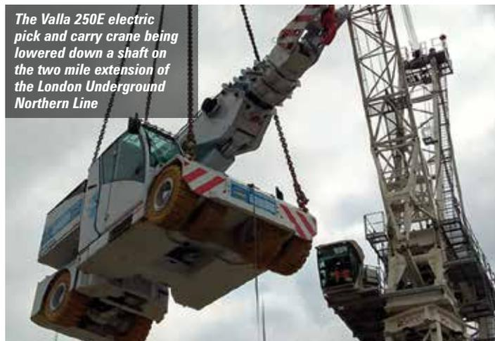
The Valla 250E electric pick and carry crane being lowered down a shaft on the two mile extension of the London Underground Northern Line
