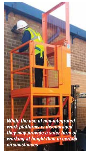
While the use of non-integrated work platforms is discouraged they may provide a safer form of working at height than in certain circumstances
