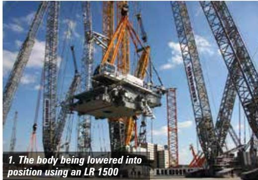
**1. The body being lowered into position using an LR 1500**
