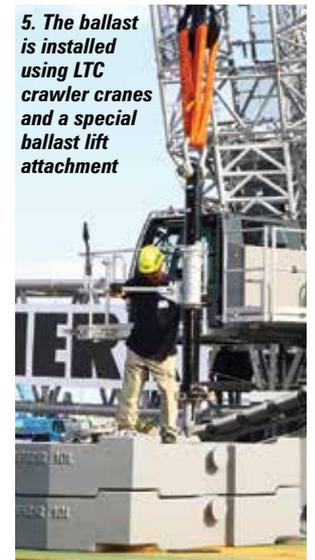
5. The ballast is installed using LTC crawler cranes and a special ballast lift attachment
