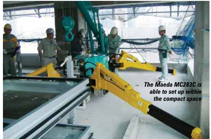
The curtain walling panel almost in place
