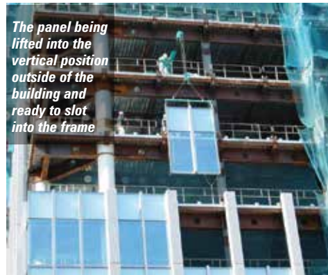
The curtain walling panel almost in place
