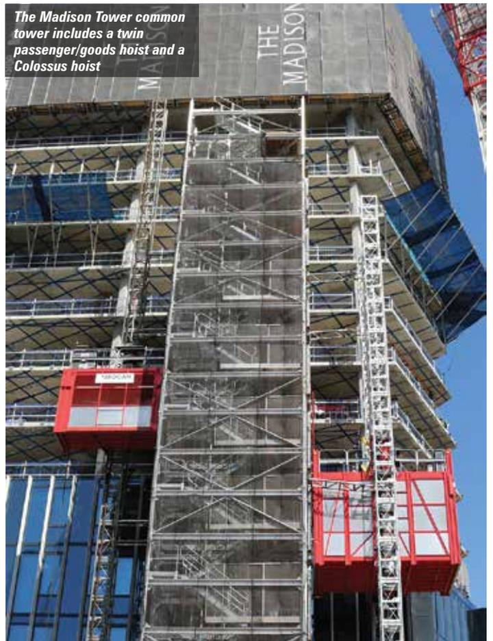
Balfour Beatty's façade manager on the project Jack Bird says: "The Madison project has two large programme critical components - the bathroom pods and the curtain wall stillages - both of which must be transported vertically and distributed to the floor plate by the Colossus hoist which has been specifically sized to ensure the largest pods - measuring 2.7 by 2.8 by 2.55 metres - can be delivered safely to site."
