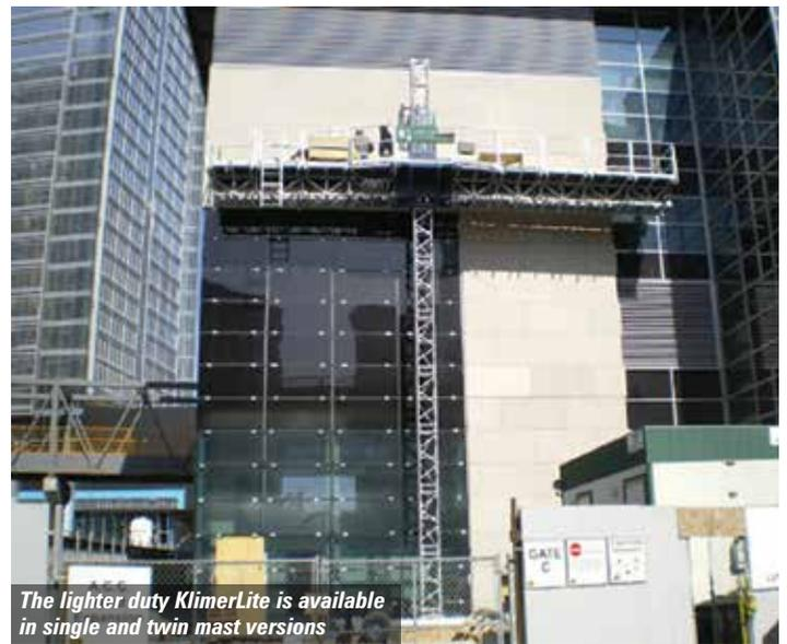
*The lighter duty KlimerLite is available in single and twin mast versions*
