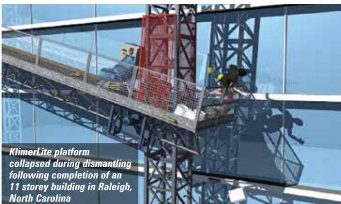
*KlimerLite platform collapsed during dismantling following completion of an 11 storey building in Raleigh, North Carolina*
