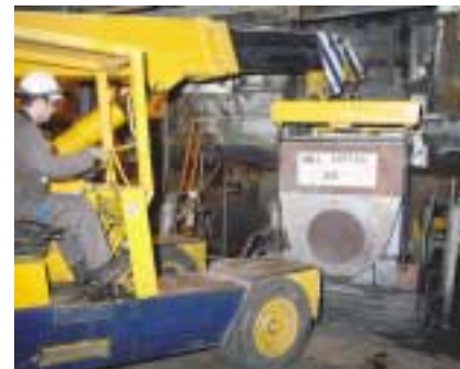
A Valla demonstrates a tough restricted headroom lift at Drax power station
