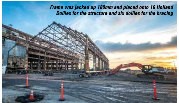
The 175 tonne steel building frame was moved almost 40 metres as part of the Pier 70 regeneration project in San Francisco
