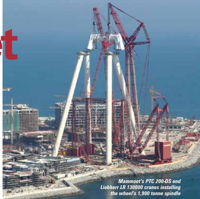
Mammoet's PTC 200-DS and Liebherr LR 130000 cranes installing the wheel's 1,900 tonne spindle
