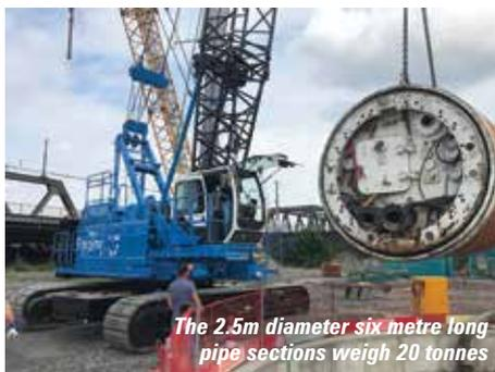
*The 2.5m diameter six metre long pipe sections weigh 20 tonnes*
