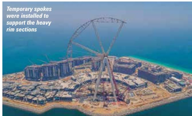
Temporary spokes were installed to support the heavy rim sections
