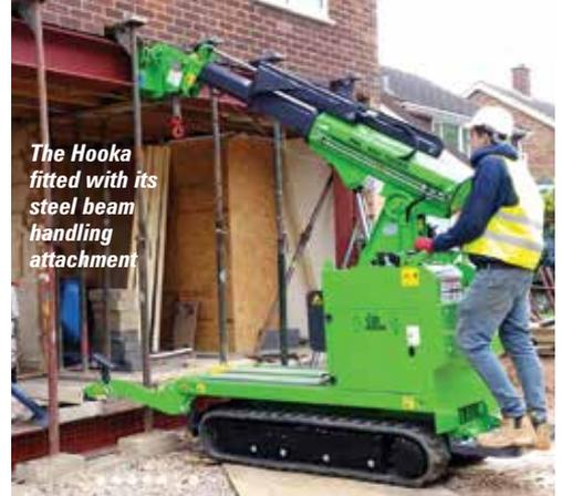
The Hooka fitted with its steel beam handling attachment
