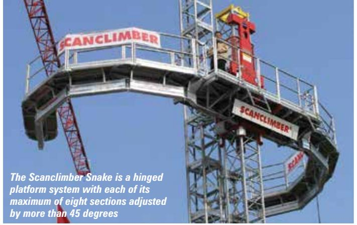
*The Scanclimber Snake is a hinged platform system with each of its maximum of eight sections adjusted by more than 45 degrees*
