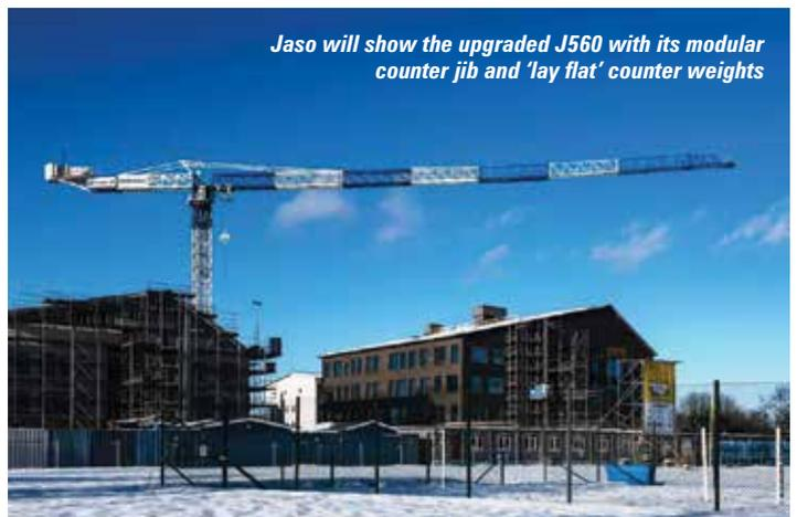
*Jaso will show the upgraded J560 with its modular counter jib and 'lay flat' counter weights*
