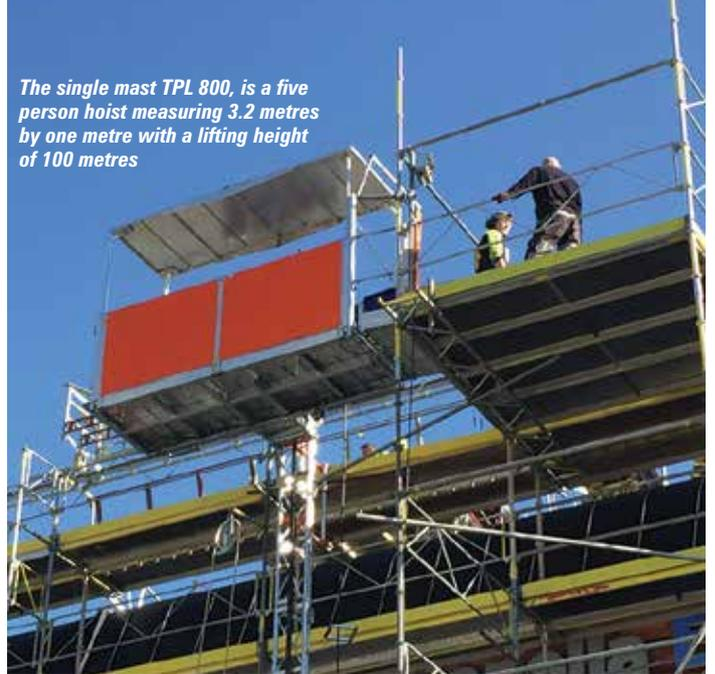
passenger mode and double that for materials. One advantage is the possibility to open the 3.2 metre platform side with bi-folding doors for loading and unloading purposes. The enhanced mast design allows tie distances of up to 7.5 metres to be achieved, giving the ability to span three storeys of a building or scaffold. The tie pipes are fixed on the mast sections via a double frame arrangement giving greater rigidity to the masts whilst still being quick and simple to install.
