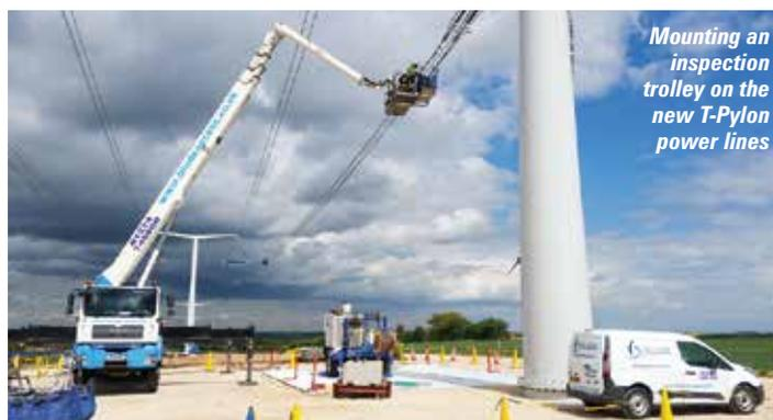
*Mounting an inspection trolley on the new T-Pylon power lines*
