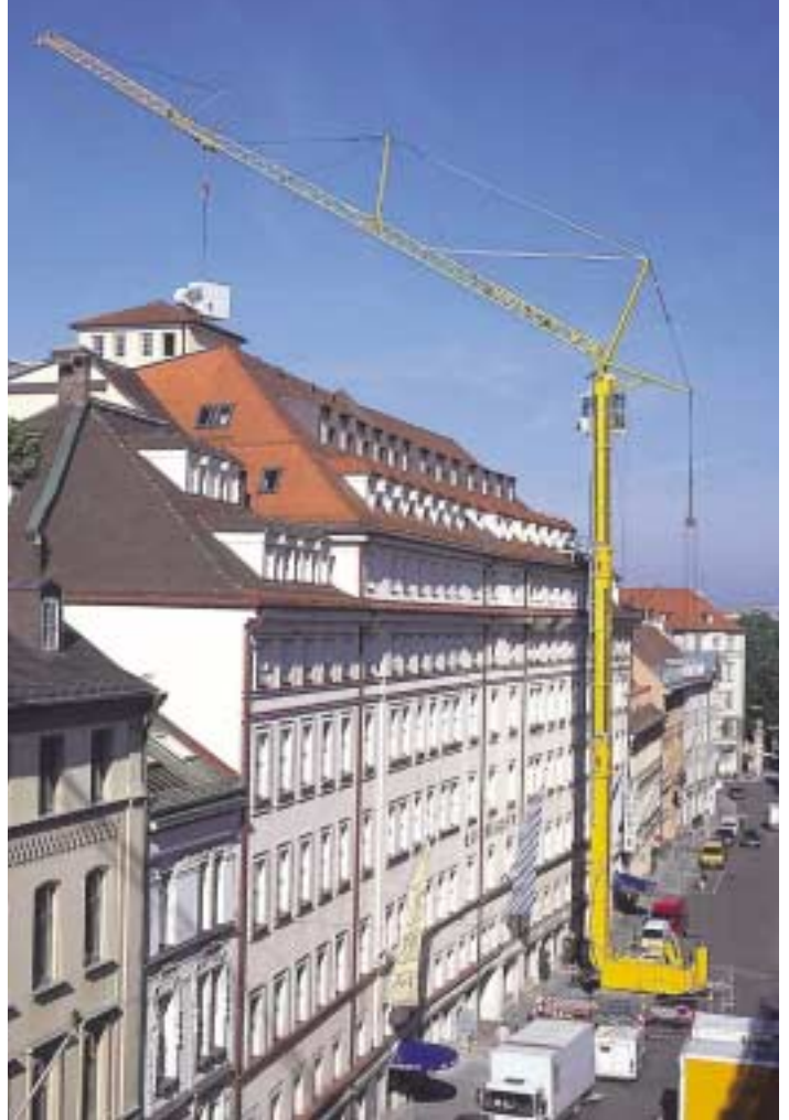
Liebherr MK100 demonstrates its up and over capability in a busy street.
