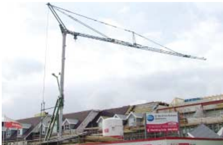
This three storey development is an ideal project for a self erecting tower crane.
