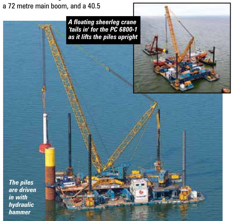
A floating sheerleg crane 'tails in' for the PC 6800-1 as it lifts the piles upright
