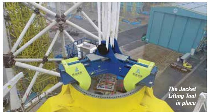
*The Jacket Lifting Tool in place*
