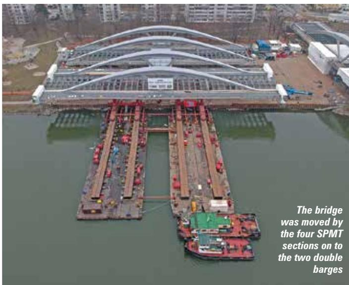
*The bridge was moved by the four SPMT sections on to the two double barges*
