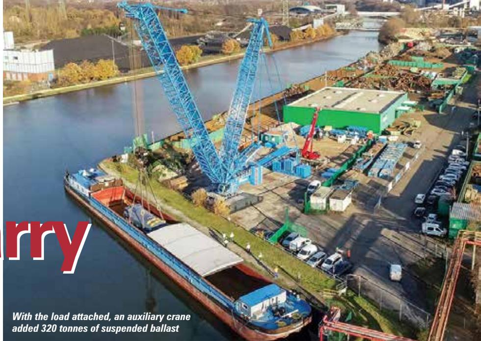
With the load attached, an auxiliary crane added 320 tonnes of suspended ballast
