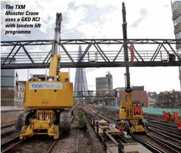
overpass. The 'Monster Crane' lifted each structure from a tractor trailer at a safe location and then carried the load along the line with a one in twenty gradient, while trains continued to travel at full speed on the adjacent line. This enabled the job to be completed in 12 weeks. The traditional solution would have involved a 400 tonne crane lifting the loads across the tracks, requiring it to be shut to trains. The severe limits on the time available for closing lines would
