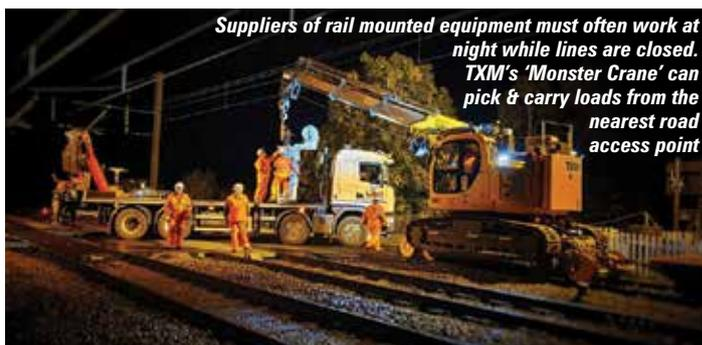
Suppliers of rail mounted equipment must often work at night while lines are closed. TXM's 'Monster Crane' can pick & carry loads from the nearest road access point
