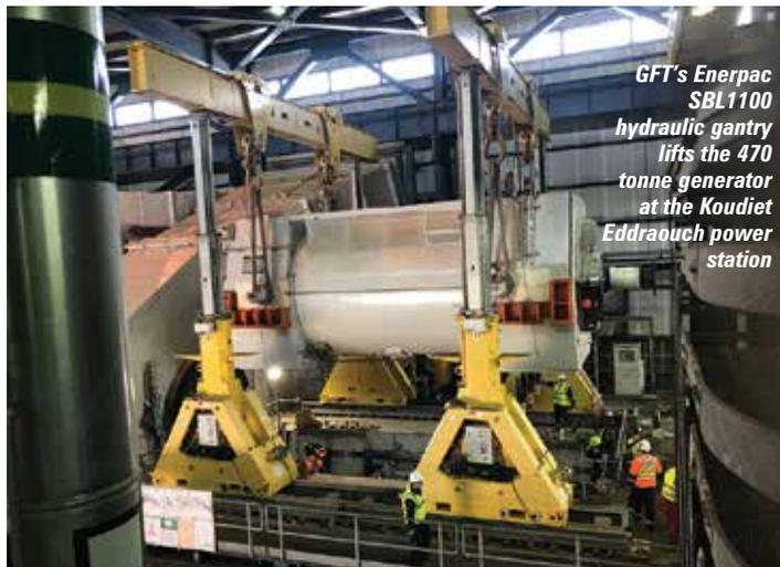
GFT's Enerpac SBL1100 hydraulic gantry lifts the 470 tonne generator at the Koudiet Eddraouch power station
