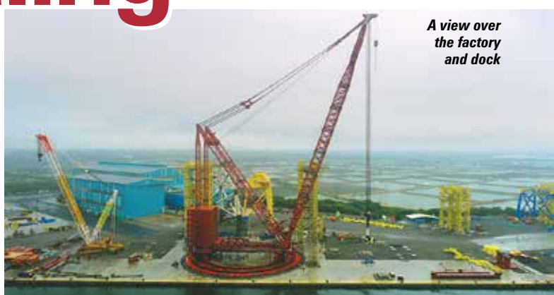
The PTC200-DS lifting a jacket with the Jacket Lifting Tool
