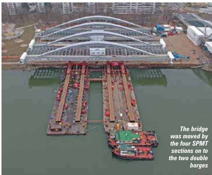
The barges were rotated 90 degrees and floated to the piers
