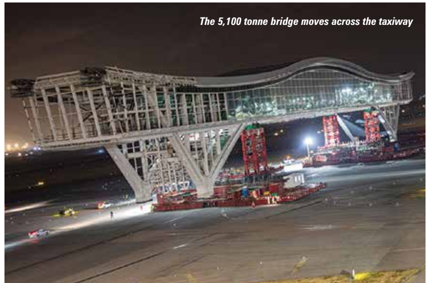
The bridge is moved into place
