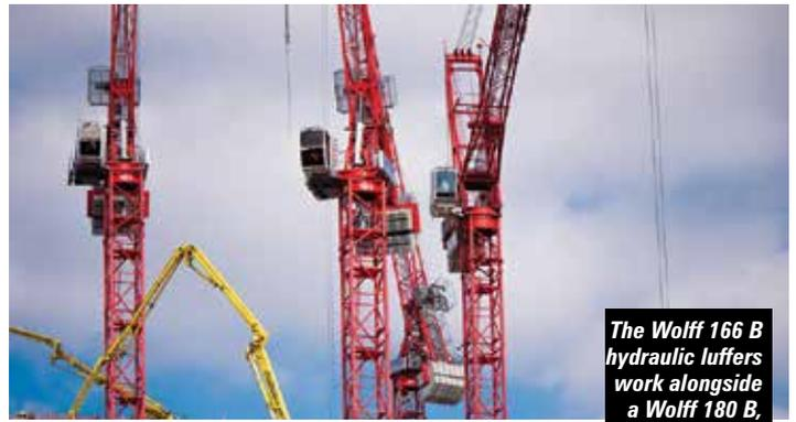
*The Wolff 166 B hydraulic luffers work alongside a Wolff 180 B, which will later be used to dismantle the smaller cranes*
