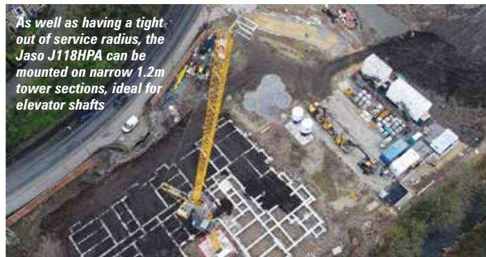
*As well as having a tight out of service radius, the Jaso J118HPA can be mounted on narrow 1.2m tower sections, ideal for elevator shafts*
