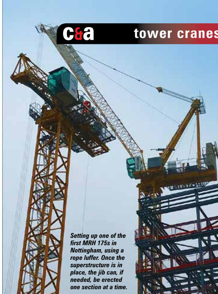
Setting up one of the first MRH 175s in Nottingham, using a rope luffer. Once the superstructure is in place, the jib can, if needed, be erected one section at a time.
