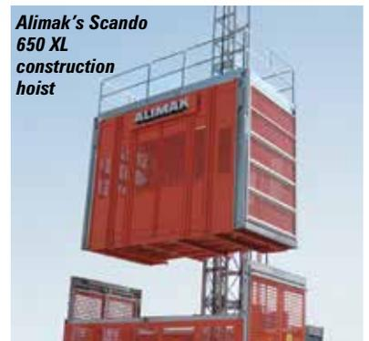
Alimak's Scando 650 XL construction hoist
