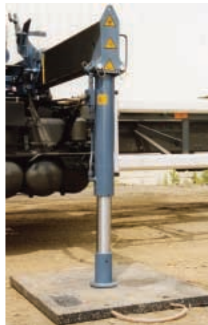
Recycled polyethylene pads provide a good foundation of known sizes and density.
