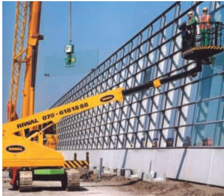
Aichi booms are being used on Holland's motorways to install sound suppression a number of the units have special 4x1m platforms.
