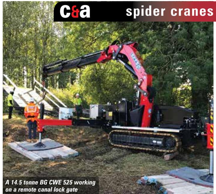
A 14.5 tonne BG CWE 525 working on a remote canal lock gate
