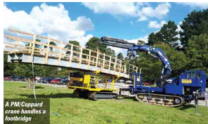
One of Hüffermann's cranes, a Palfinger on a wheeled chassis
