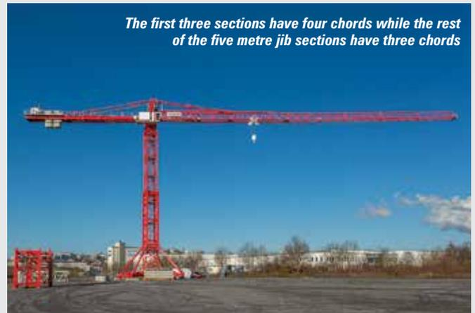
The first three sections have four chords while the rest of the five metre jib sections have three chords
