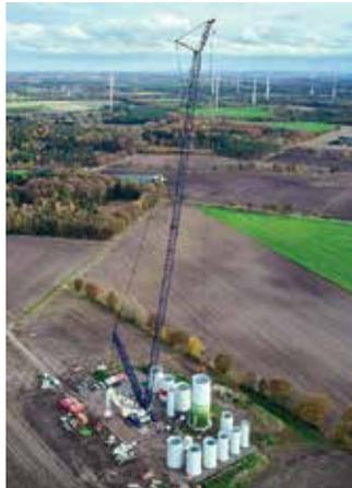
SL10DF2BV wind power boom system. The 168 metre main boom and fixed offset jib of up to 24 metres provides hook heights up to 192 metres with a capacity of 110 tonnes. Features include Liebherr's VarioTray and V-Frame ballast systems.
