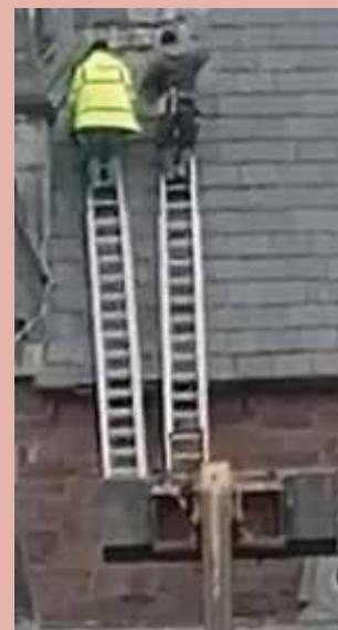
Spotted just before Christmas, three men repairing damage to the roof of St John's Church in Tralee, Ireland, following Storm Barra. To reach the roof they combined a telehandler fitted with a material bucket with two long ladders - right in the middle of the busy town centre!
