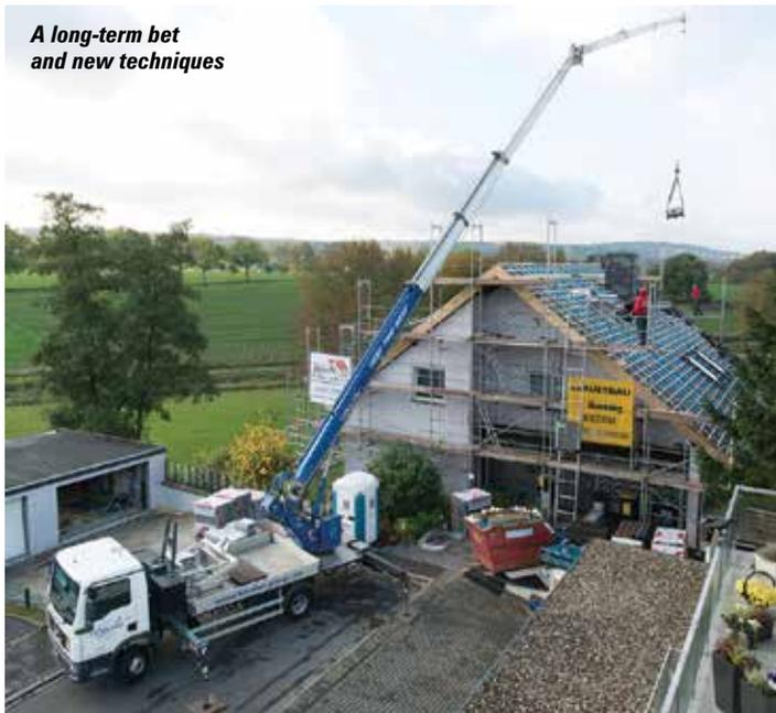
counterweight within 12 tonne axle loads. Maximum radius is 38 metres where it can lift 800kg at a height of 22 metres.
