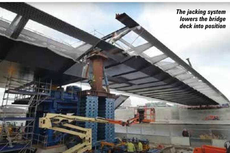
The jacking system lowers the bridge deck into position
