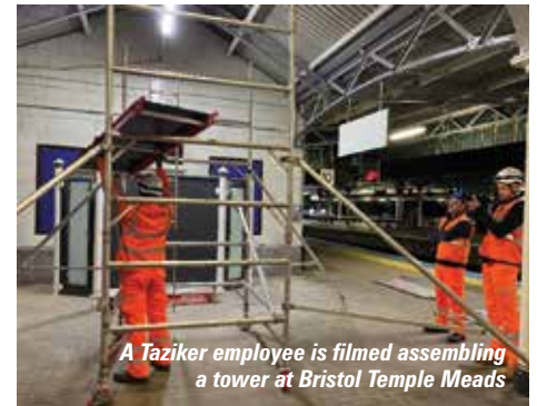
Three were needed to safely assemble a tower in this location
