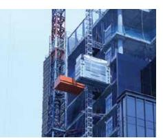
management and diagnosis, a lateral door option and being able to configure the hoist. A new square mast - the M650 - has been designed which has the capacity for two hoists, doubling the load capacity and allowing operators to work on different floors.
