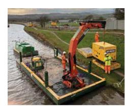
waterway bed. This set-up is similar to ocean going 'jack up vessels', in which the jacks can lift the boat out of the water but is only possible at pre-set inboard spacings. Outrigger type legs excel in providing a wide footprint for good lateral stability. However, unlike their vertical counterparts, they cannot be used to lift boats out of the water."
