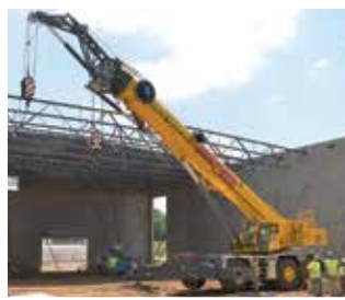
The GRT9165 with jib installed
