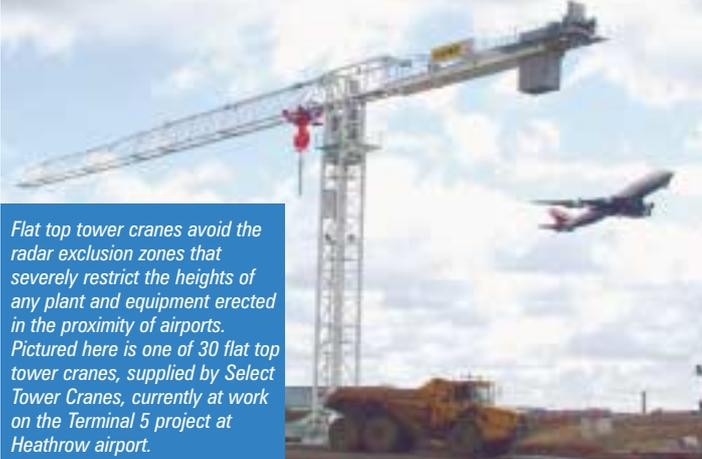
Flat top tower cranes avoid the radar exclusion zones that severely restrict the heights of any plant and equipment erected in the proximity of airports. Pictured here is one of 30 flat top tower cranes, supplied by Select Tower Cranes, currently at work on the Terminal 5 project at Heathrow airport.
