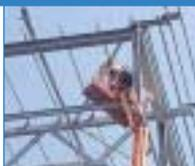
A worker was seriously injured last month when the ground gave way under a JLG 600AJ articulated boom lift working on the new Joseph Wright sixth form building at the Derby College. The machine fell against the building's framework, which prevented it from falling further.
