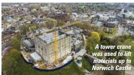
Fixing the steel beams in place at Norwich Castle
