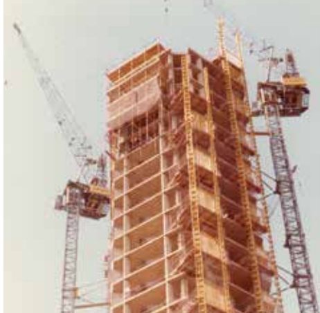
Three of Laing's 50HBs were used to build the Penta Hotel in Cromwell Road, London
