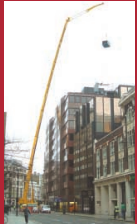
NMT recently put its new Demag AC200-1 to the test when it was used to lift a number of air conditioning units onto a roof in central London for Mechanical Movements. The crane fully utilised its 68 metre main boom with a 17 metre fly-jib set at 40 degrees.
