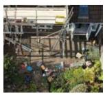
found that the company failed to plan, manage or monitor work at height, and provide adequate scaffolding or an appropriate means to transport materials to the roof.
