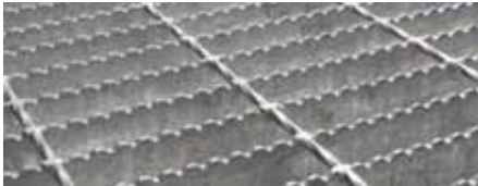
The common serrated grating is a 'wavy' style which is very smooth so when wet can become extremely slippery
