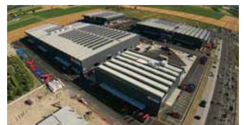
Magni completed its current facility expansion in May 2021 enabling it to double the number of machines
